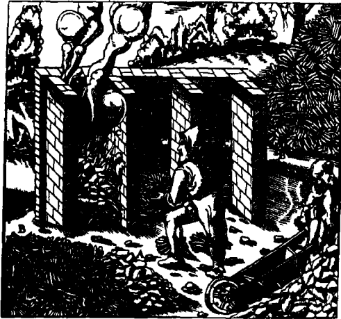
Fig 63 Roasting copper matte (after AGRICOLA, de re Metallica )
