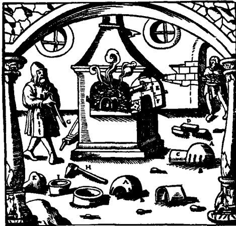
Fig. 47. Refining silver by cupellation (after AGRICOLA, de re Metallica )
