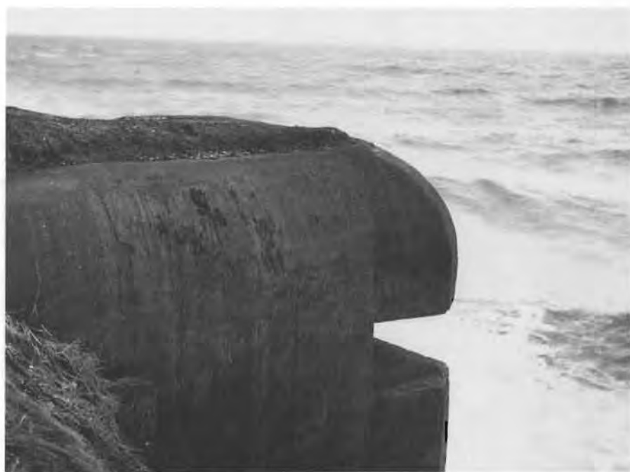
BUNKER WITH TWO EMBRASURES: THIS TYPE OF FORTIFICATION IS RARE ON ACCOUNT OF MULTIPLE CONCEALMENT PROBLEMS
