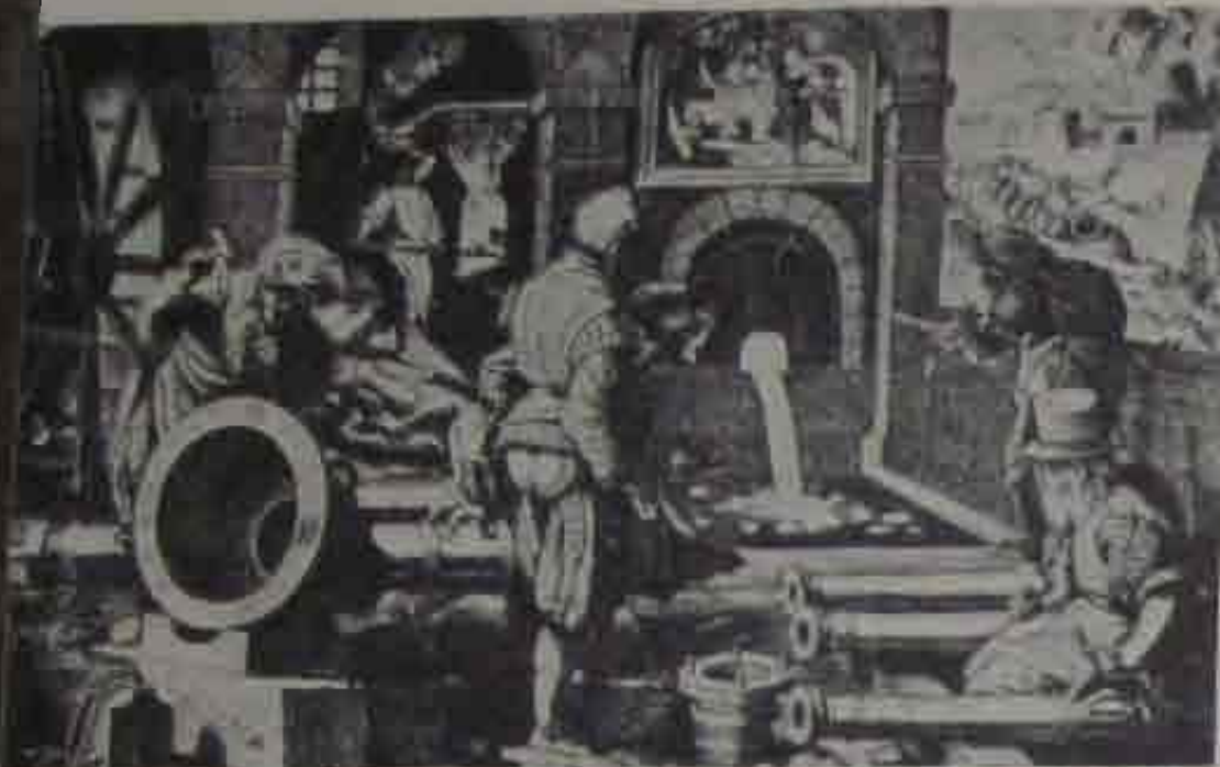
1: Sixteenth century cannon foundry, showing fortification and cannons in action in the background. The heavy demand on the mining industries that followed the introduction of cannon in the fourteenth century was likewise registered in the necessary expansion of finance. Here lies the beginning of the cycle of mining, mechanization, munitions, and finance: more dangerously evident today than ever.
