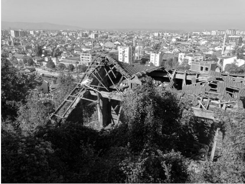
Figure 8.9 A view over the city of Prizren, with a residence gutted and destroyed during the 2004 anti-Serb pogrom.
