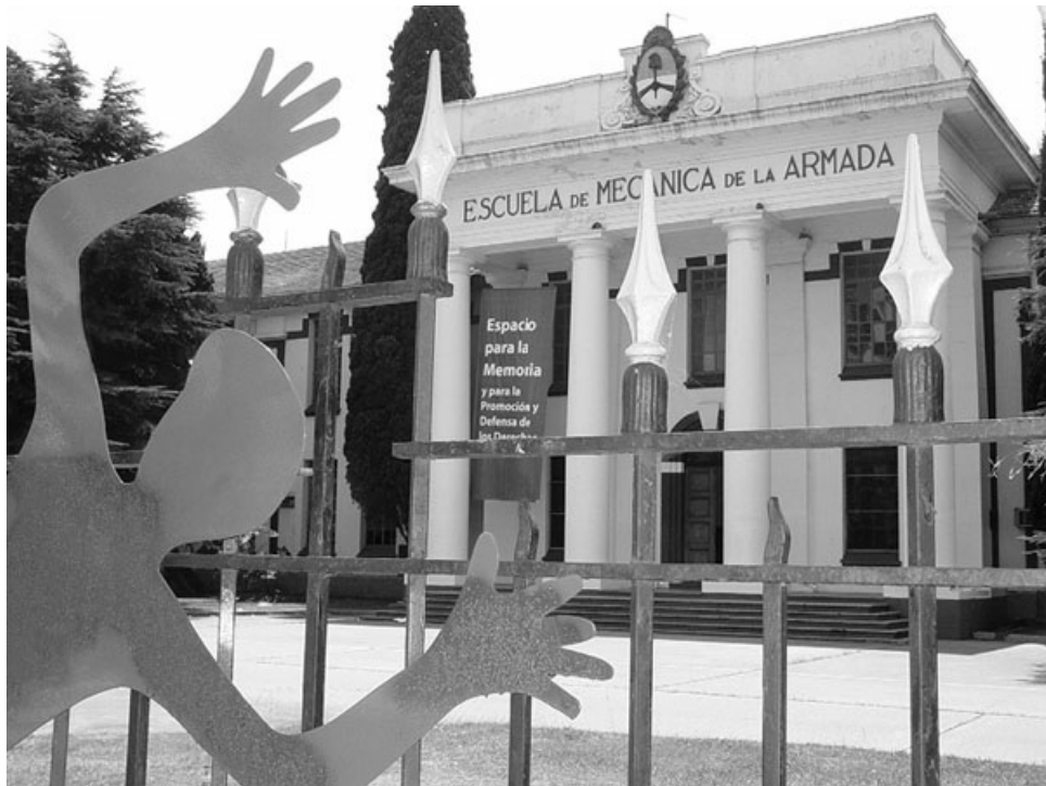
Figure 14.5 The façade of the Escuela Mecánica de la Armada (Naval Mechanics School) in Buenos Aires, Argentina. A principal detention and torture center during the years of military dictatorship (1976–1983), its operations gave rise to the largest-ever trial of accused perpetrators of atrocity crimes under the junta —sixty-eight former officials in all.
