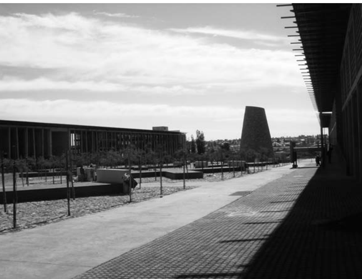
2 View across the Walter Sisulu Square of Dedication, 2005. Designed by Studiomas, the winners of the architectural competition. Photo by Lindsay Bremner
